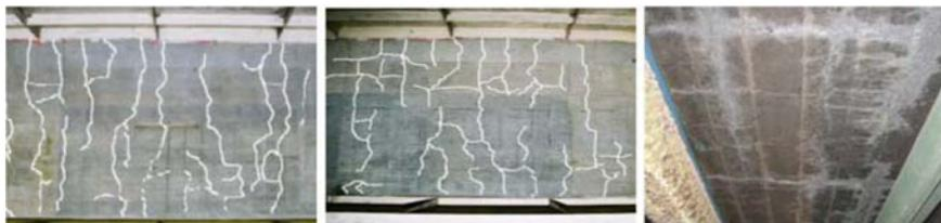
(a) 1Direction Cracks (b) 2 Direction cracks (c) 2Direction cracks and Free lime
