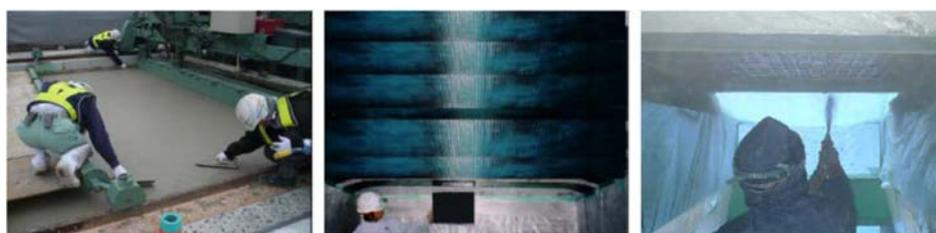
(a) SFRC overlay (b) CFS bottom side Reinforcement (c) spraying method of mortar
