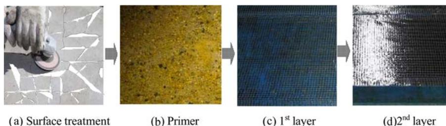
**Fig. 6.** Adhesion processing of CFS.
