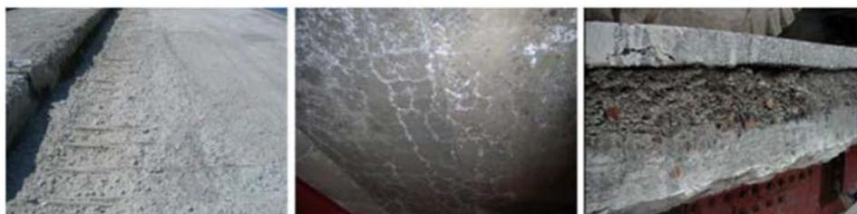
(a) scaling (b) Cracks and Free lime (c) gravel of internal
