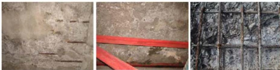
(a) Rebar leakage (b) Deposition of rust (c) Rebar leakage and Rust
