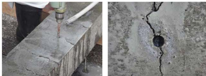
Fig. 6. Drilling of reinforced concrete cracks.
