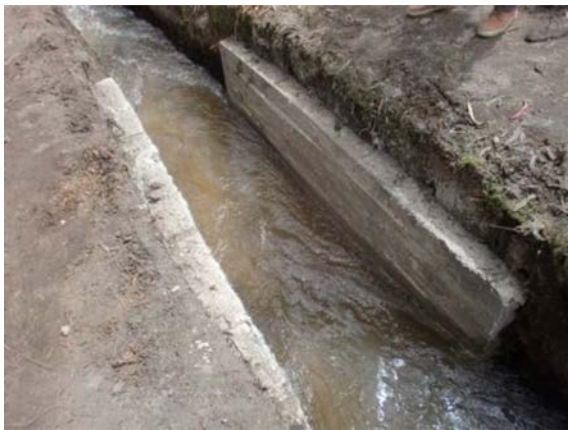
Fig. 2. Canal section casted with self-healing concrete (with bacteria) under working conditions only 5 days after casting.
