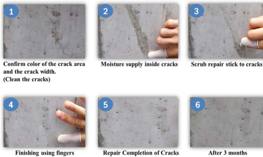
Fig. 24. New repairing method for micro-crack of concrete [adapted from T.H Ahn et al. 2014, 2015].
